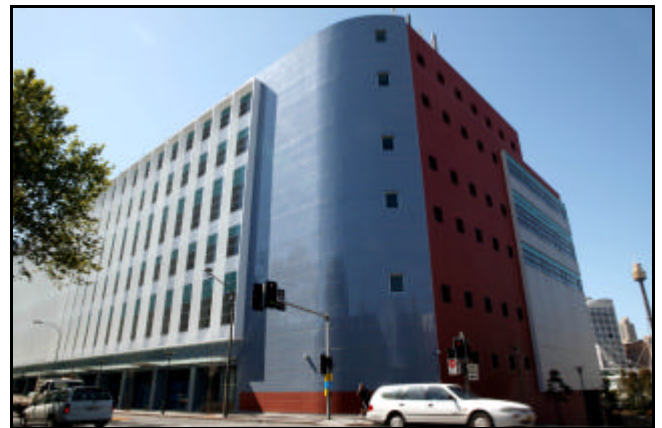
ac3's second data centre is located within Global Switch, on the outskirts of the CBD.
